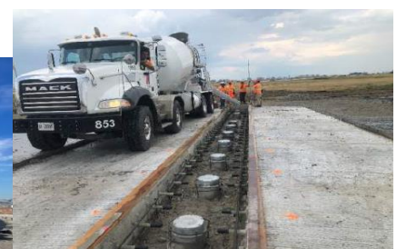
Stage 1C: Pouring concrete for Taxi D2 stop bar.
