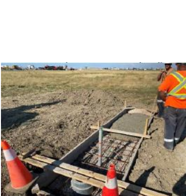
Stage 1D: Pouring the guidance signs base on Taxiway D3.
