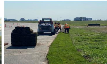
Stage 1C: Placing sod at Taxiway D1 along asphalt edge
