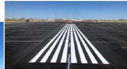
Stage 1D: Runway centreline markings at Taxiway D3 intersection (1 st coat)
