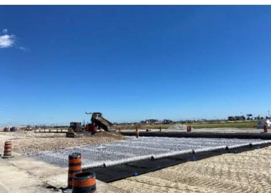
Stage 2C: Placement of granular base and installation of geotextile and geogrid.
