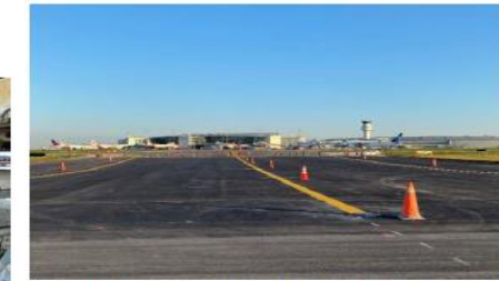
Stage 1D: Taxiway D3 centreline and double yellow edge markings painted.
