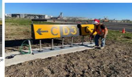
Stage 1D: Installing old D3 sign on new guidance sign base.
