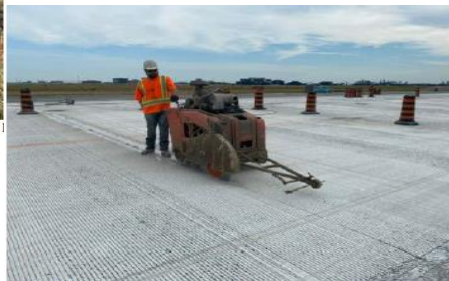
Stage 1C: Relief cuts on new PCC slab joints.
