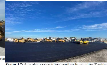
Stage 1C: 6 asphalt spreaders paving in escalon Taxiway D1.
