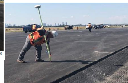
Stage 1C: Surveyor marking vertices of concrete slabs below asphalt for routing and sealing.
