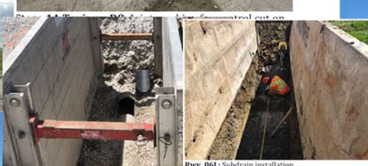
Rwy. 06L: Subdrain installation.
