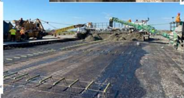
Stage 1B and 1E: Filter cloth, geogrid and granular base installation.
