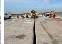
Stage 1E: Trenching for electrical conduits.
