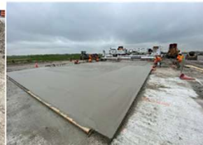
Stage 1A Taxiway D8: Surface PCC concrete paving.
