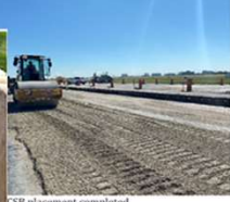
CSB placement completed.
