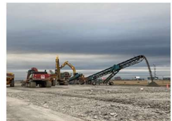
Concrete crushing operation commenced on RWY 06L-24R.
