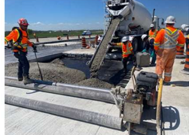
Stage 1A: Pouring concrete slab on Runway
