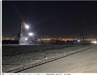
Two breakers at work on RWY 06L-24R
