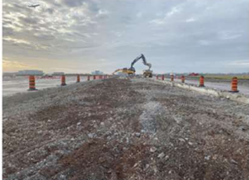
Excavating concrete on TWY D8 and hauling to crusher.
