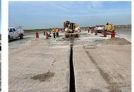
Stage 1E: Trenching for electrical conduits.
