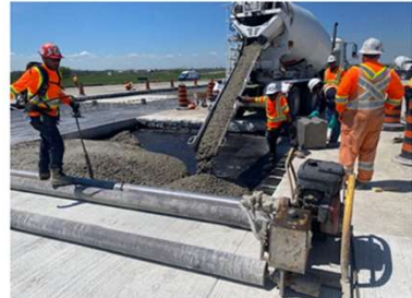
Stage 1A: Pouring concrete slab on Runway
