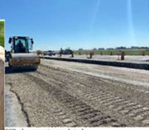
CSB placement completed.
