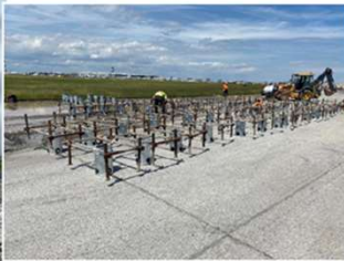
Stage 1E: Trenching for electrical conduits.
