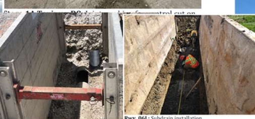
Rwy. 06L: Subdrain installation.
